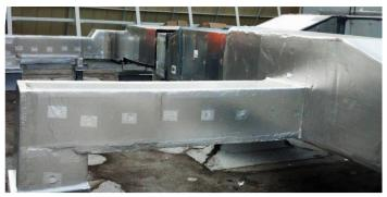
**PRO TIP:** To cover washers, cut out squares of jacketing at approx 6". Adhere the patches over the washers. Squeegee in place.
